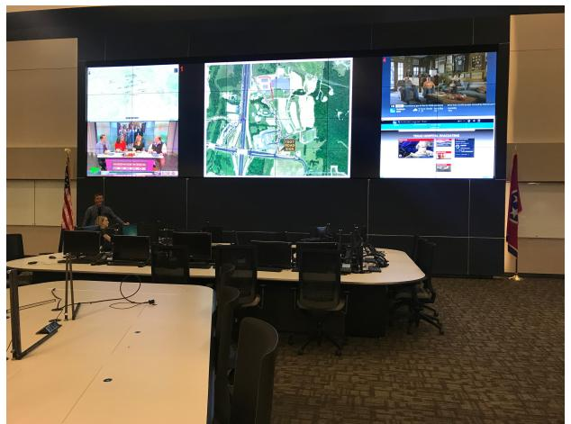
Planar Clarity Matrix 8x4 LED Video Wall with Planar VCS Windowing Processor, Crestron DM Video Distribution and Control
