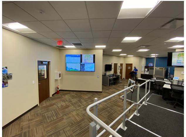
Planar Clarity 7x2, and 2x2 Clarity Matrix LED Video Wall, Crestron DM Video Distribution and Control
